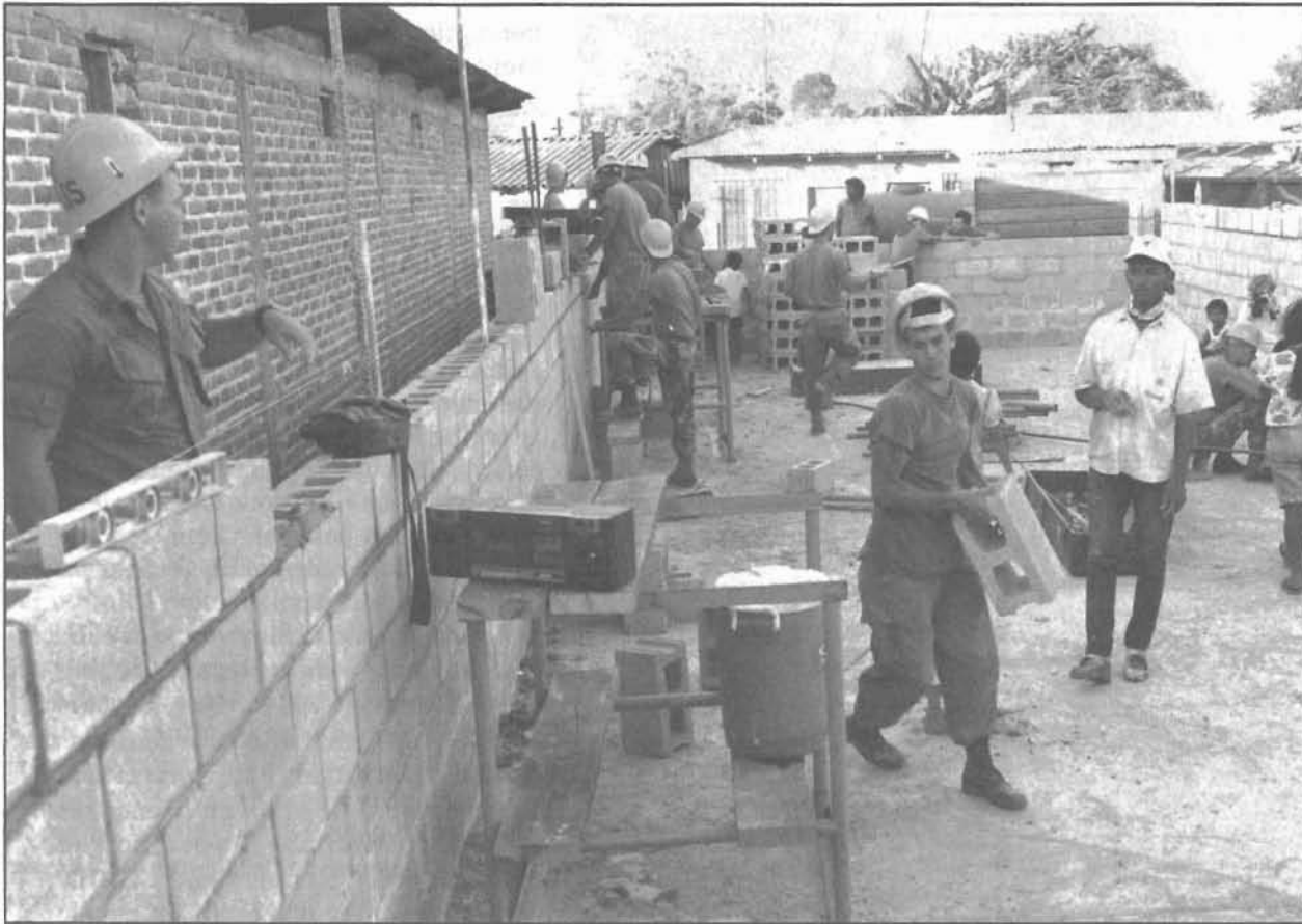
National Guard engineers work on a block wall during construction of a school in Comayagua, Honduras .
