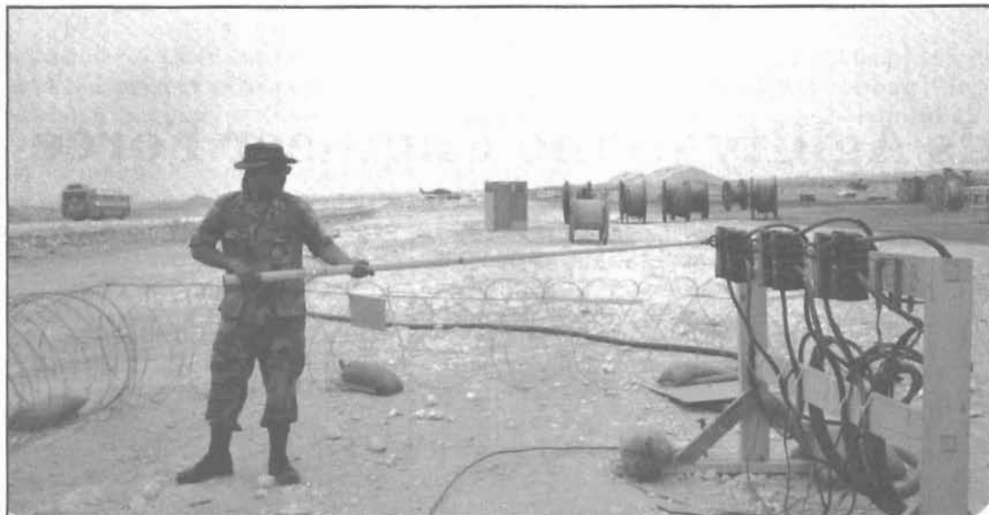
Prime power team member Sergeant Sidi Hassaneodin opens a fused disconnect on a medium voltage distribution network.
