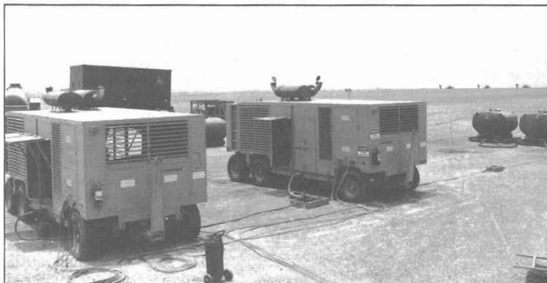
The prime power plant at the west heliport, Dhahran Airbase, Saudi Arabia. Each generator produces 750 kilowatts.
