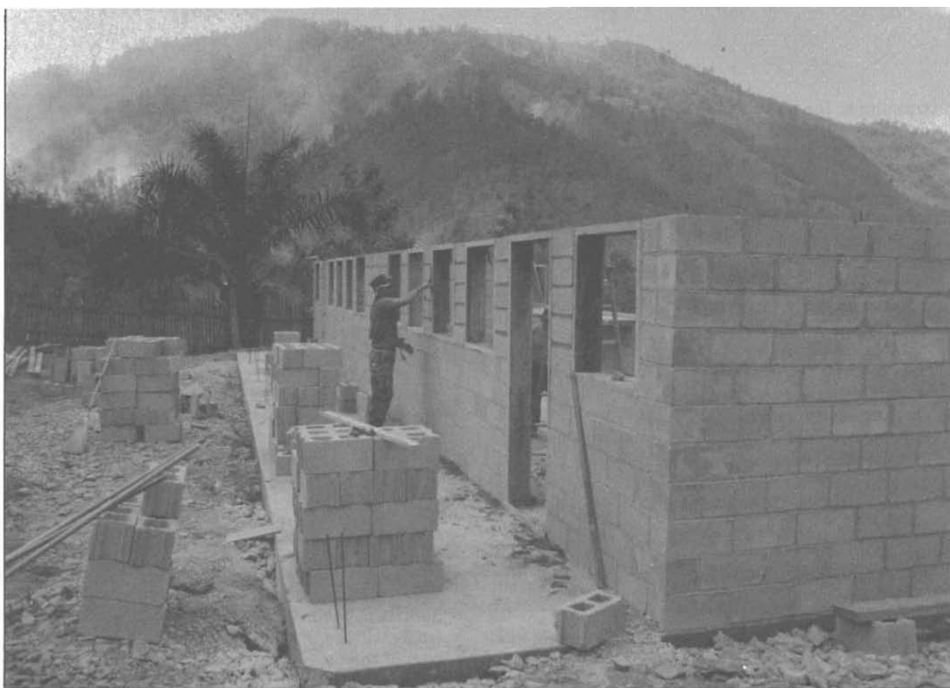
An engineer finishes placing window frames in a new school building in Macora, Honduras.
