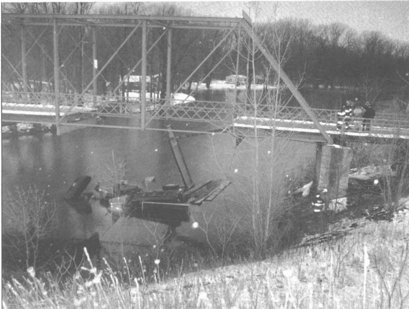
Haiti Island Bridge the morning of November 13, 1990, the day after its failure. Forty feet of roadway collapsed into the Seneca River when a snowplow struck one of the bridge's vertical beams. Note the partially submerged plow. (Photo by Craig Jackson, by permission of Syracuse Newspapers)
