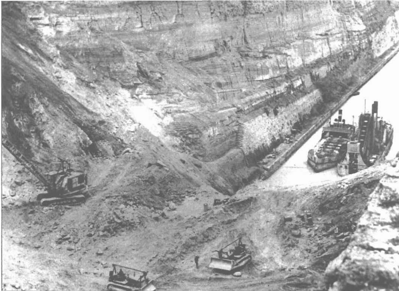
The Dredge Poseidon (right center) at work clearing the Corinth Canal. (Photo courtesy USACE Office of History, Research Collection)
