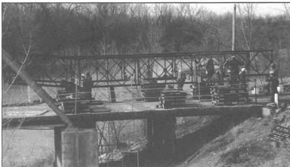
Left: Echo Company engineers begin constructing the Bailey. Note the 54-inch cribs for the nearshore rocking rollers.
