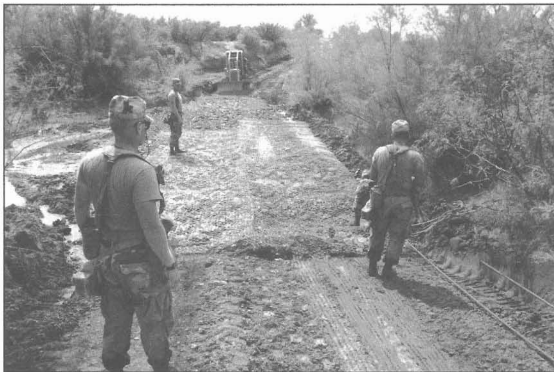
Soldiers from the 39th reinforce a dirt road after heavy rains damaged it. (Photo courtesy U.S. Border Patrol)
