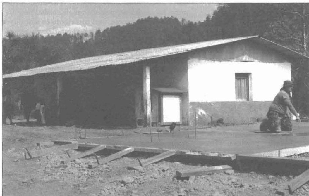
With the old school serving as a backdrop, an engineer smooths the concrete foundation for a new school in the Honduran village of El Corozo.
