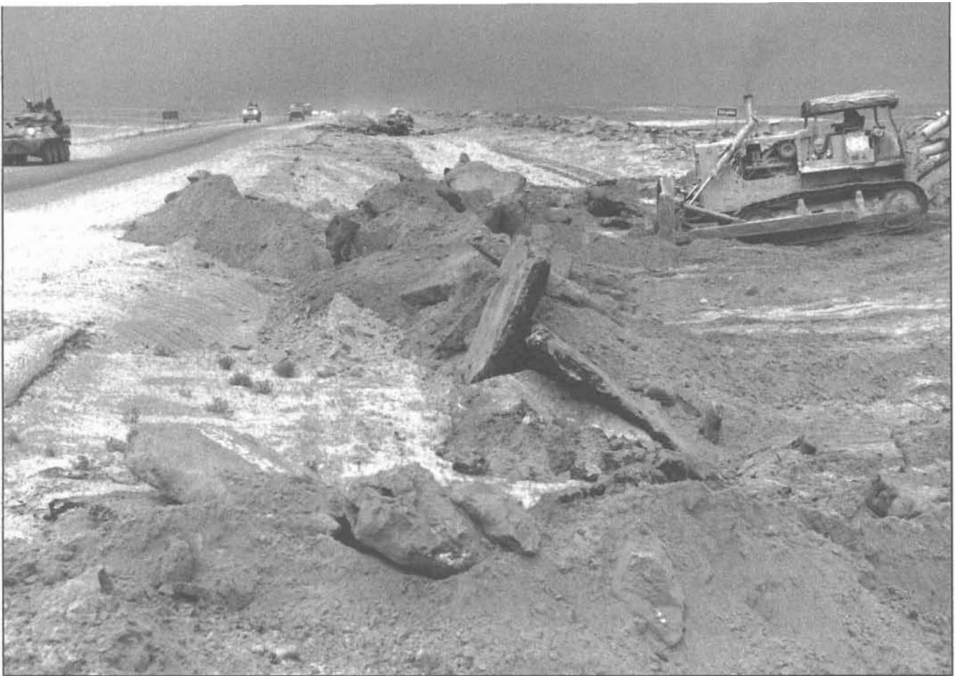
Construction crews repair Nulseeb Road near the Saudi border. (Photo by Jonas Jordan)
