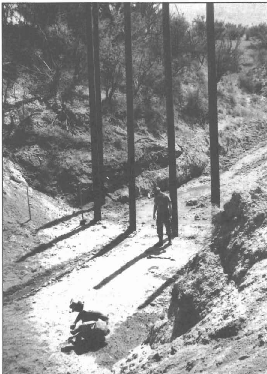
Alpha Company soldiers mark where they will place drainage tubes in a gulley. The large poles will support the tubes, forming a giant culvert. (Photo by Galen Putnam)
