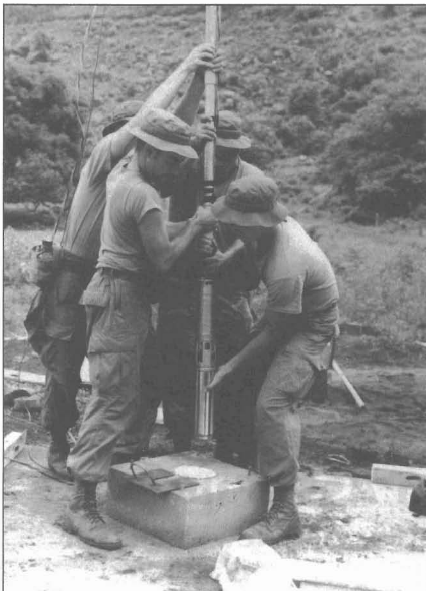
Engineers lower a submersible pump into a well casing on Tiger Island, Honduras.
